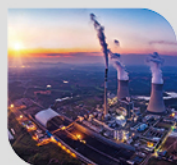
Environmentally friendly heating
