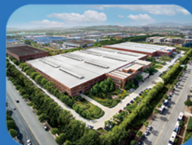
Laishan Industrial Park
